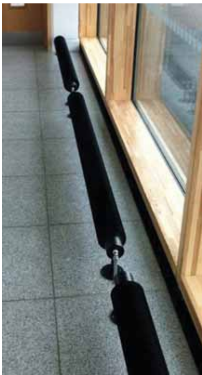
Finned tubes (to be trenched).
