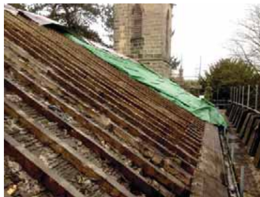
Above: St. John's in 2015 during re-roofing.
