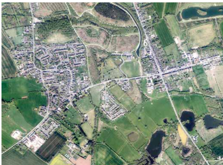
Above: the form of Donisthorpe is a legacy of coalmining; now, at the heart of the National Forest and well-connected by the A42, a new future is emerging for the village.
