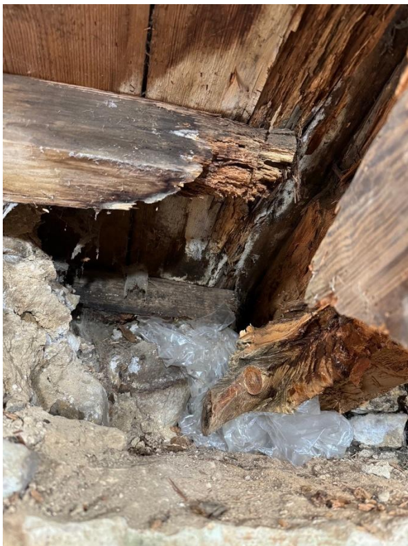
Figure 3 - Wet rot within the South Aisle beam.
