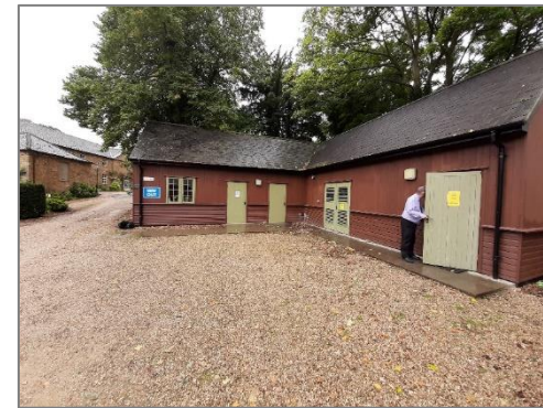
Photo 9. Potential electric vehicle (EV) charging area
