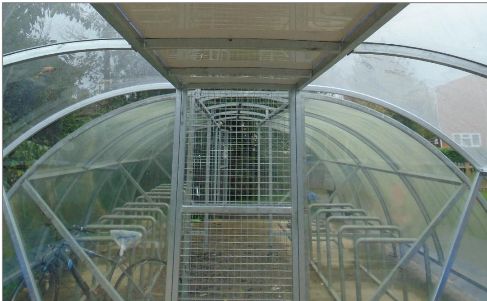
Photo 15. Lockable Internal Door
